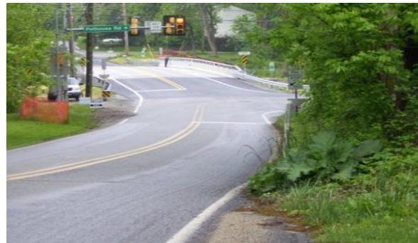
Williams Corner new bridge 2011 North from Whitehorse Road
