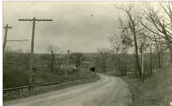
Williams Corner covered bridge 1832 North from Whitehorse
